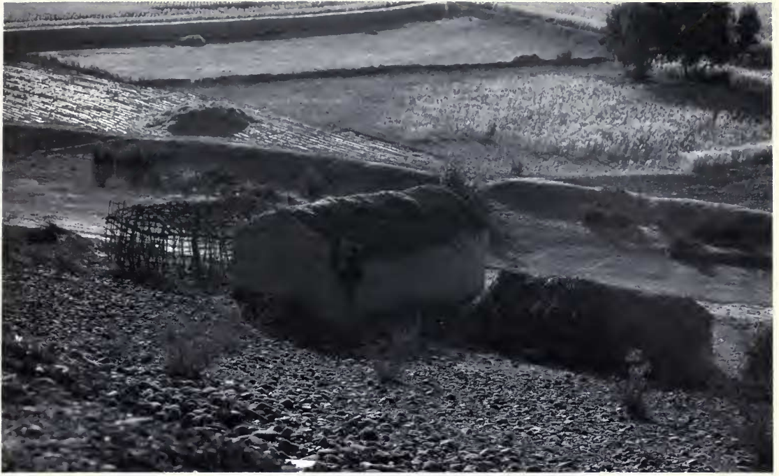
FIG. 14. Agricultural field just outside of Awaran. The roof of the building in the center is mostly made of Nannorrhops and Tamarix branches and leaves. The main support structure, visible on the building under construction to the left, consists of Tamarix timbers and heavy branches. The fields in the background contain ripening wheat. (Photo taken 10 March 1990 by S. M. Goodman.)
